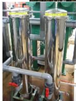
20m 3 /hr Deionised Water Treatment Plant
