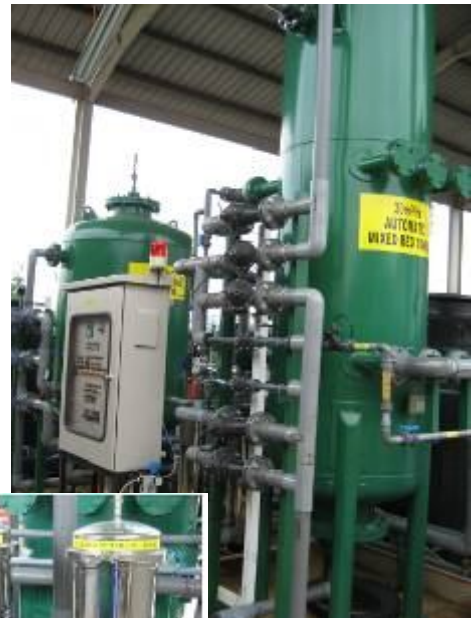
20m 3 /hr Deionised Water Treatment Plant
