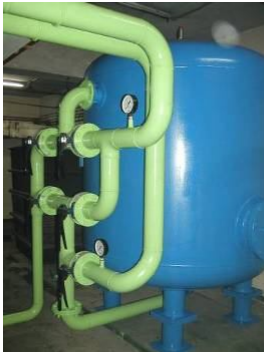
40M 3 /Hr - For Filtering Main JBA Water Supply Line
