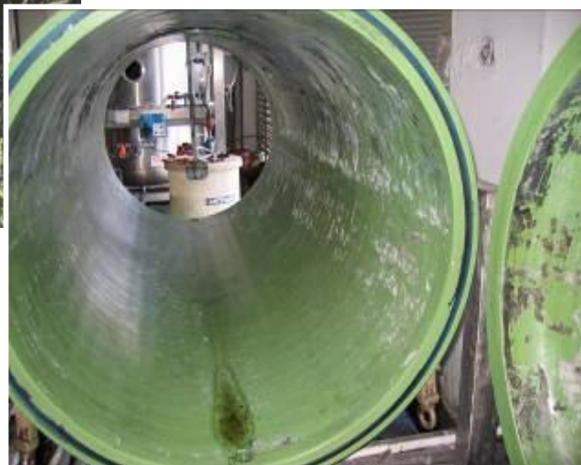
After cleaning and remove the sludge
